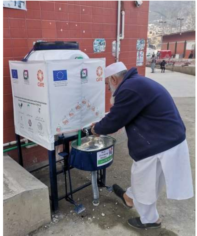
Paddle based handwashing stations installed in hospitals in Abbottabad
